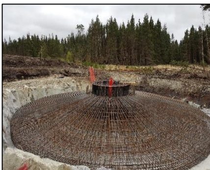
Plate 3.1 Turbine Base ‘Anchor Cage’
