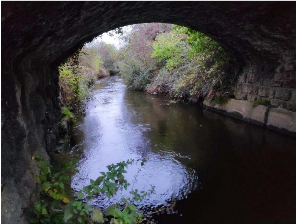
Plate 3.9 Site 9 on the Silver River at Millbrook Bridge
