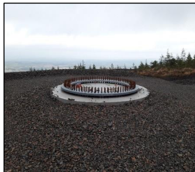
Plate 3.2 Finished Turbine Base
